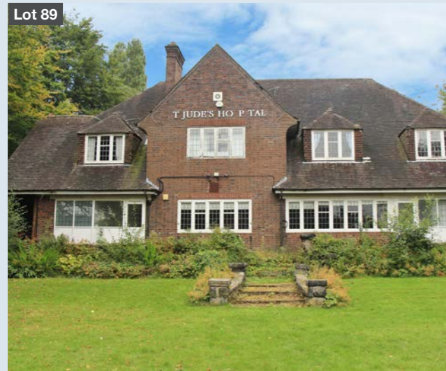
Lot 89 30 SEP Newcastle-Under-Lyme, Staffordshire £477,000 Former private clinic with potential for alternative use and / or development. VISIT WEBSITE
