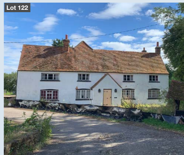
Lot 122 18 FEB Owlswick, Buckinghamshire £3,032,000 Freehold former public house with planning for nine houses. VISIT WEBSITE
