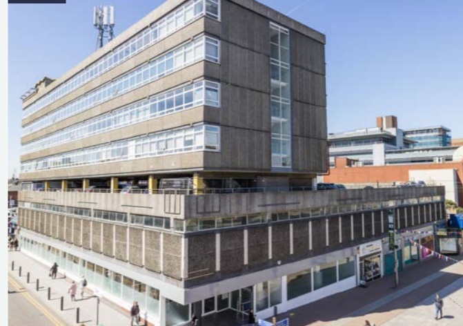
Central House, Southend-On-Sea
