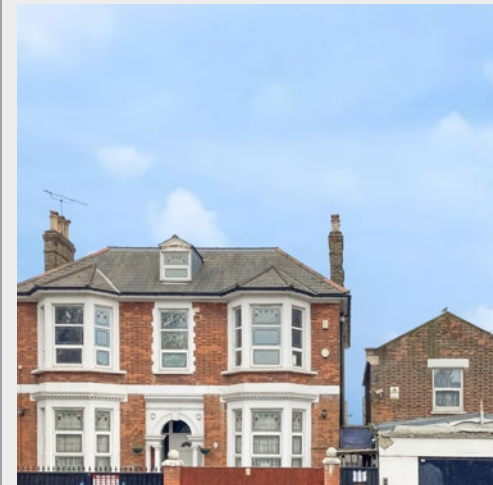
4 Woodberry Down, Finsbury Park, London, N4 SOLD AFTER AUCTION FOR IN EXCESS OF £3M Freehold site extending to approximately 942.9 sq m (10,149 sq ft). Vacant
