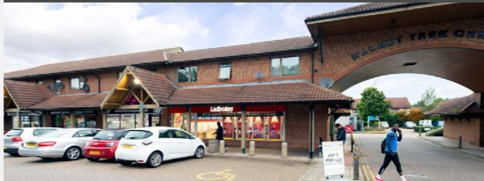
Lot 109 - Ladbrokes, Milton Keynes Betting Shop - holding over
