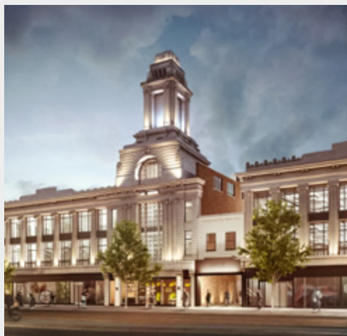
Dept W, 69-89 Mile End Road, London E1 DISPOSAL OF 55,380 SQ FT on behalf of Schroder UK Real Estate Fund. Redeveloped office let to Queen Mary University
