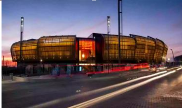
Elwick Place Retail and leisure scheme opened in Jan 2019 housing the Picturehouse Cinema with 6 state of the art screen, 9 retail / restaurants, a 58 room Travelodge and event space.
