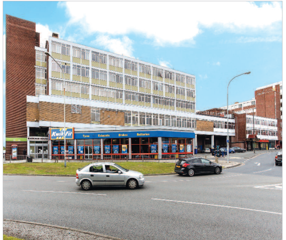
PLEASE SEE THE WEBSITE FOR MORE PHOTOGRAPHS INCLUDING AN AERIAL PHOTOGRAPH
